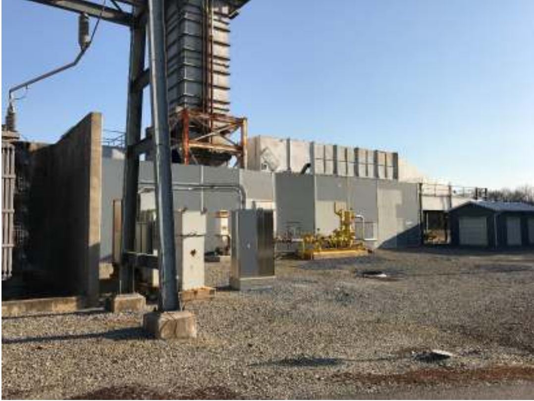
Photo 63 – VanSant Generating Station
