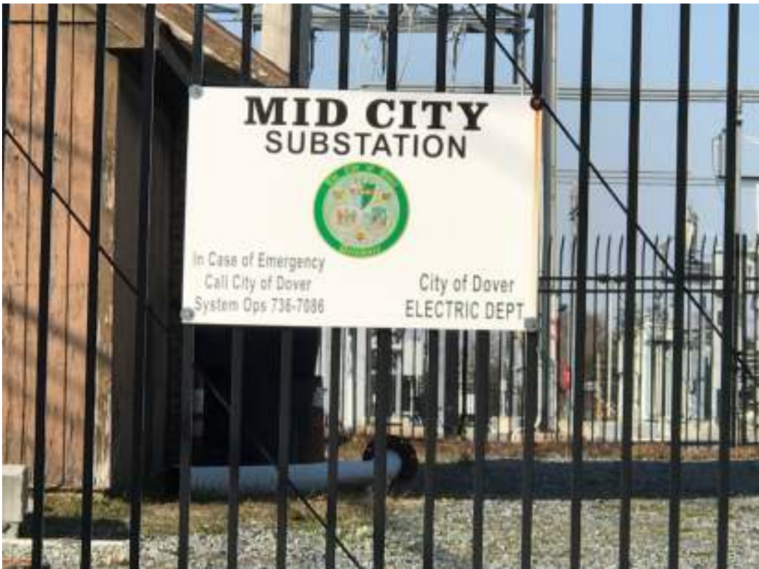
Photo 40 – Mid City Substation
