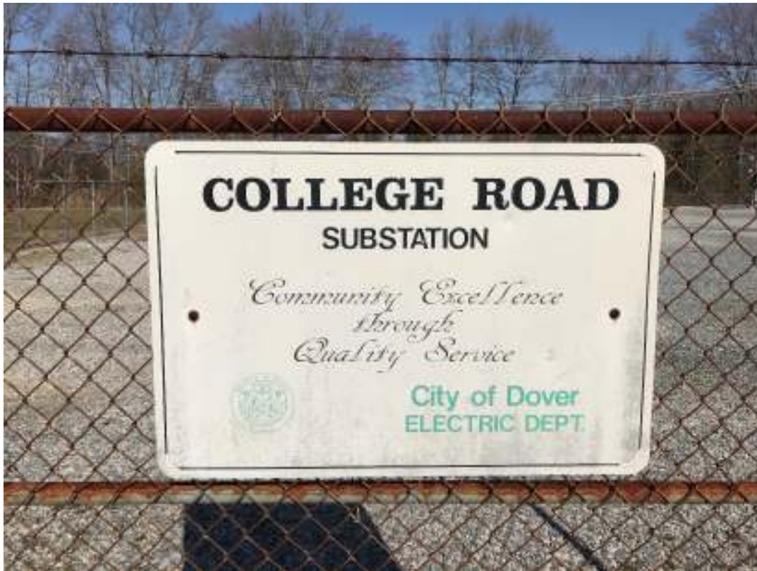
Photo 7 – College Road Substation
