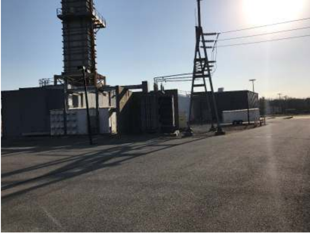
Photo 61 – VanSant Generating Station
