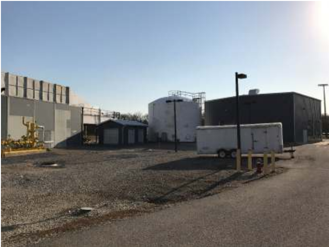
Photo 62 – VanSant Generating Station
