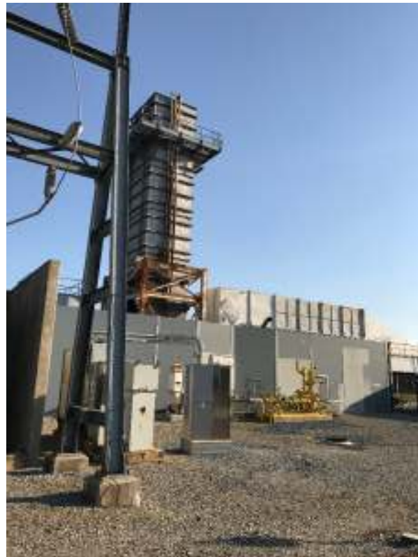
Photo 64 – VanSant Generating Station
