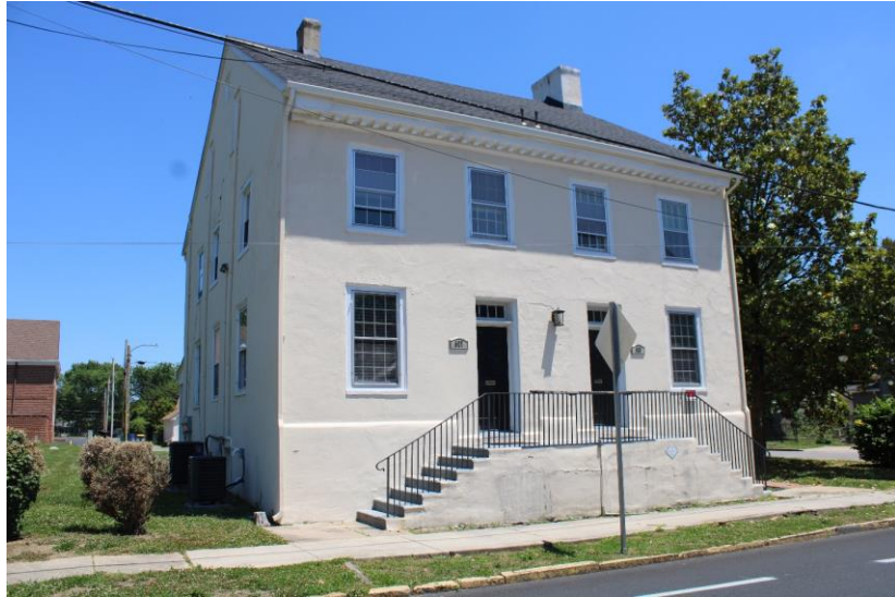
527/529 S State Street Renovation
