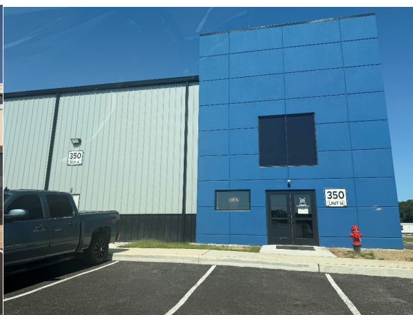
350 Lafferty Lane Warehouse
